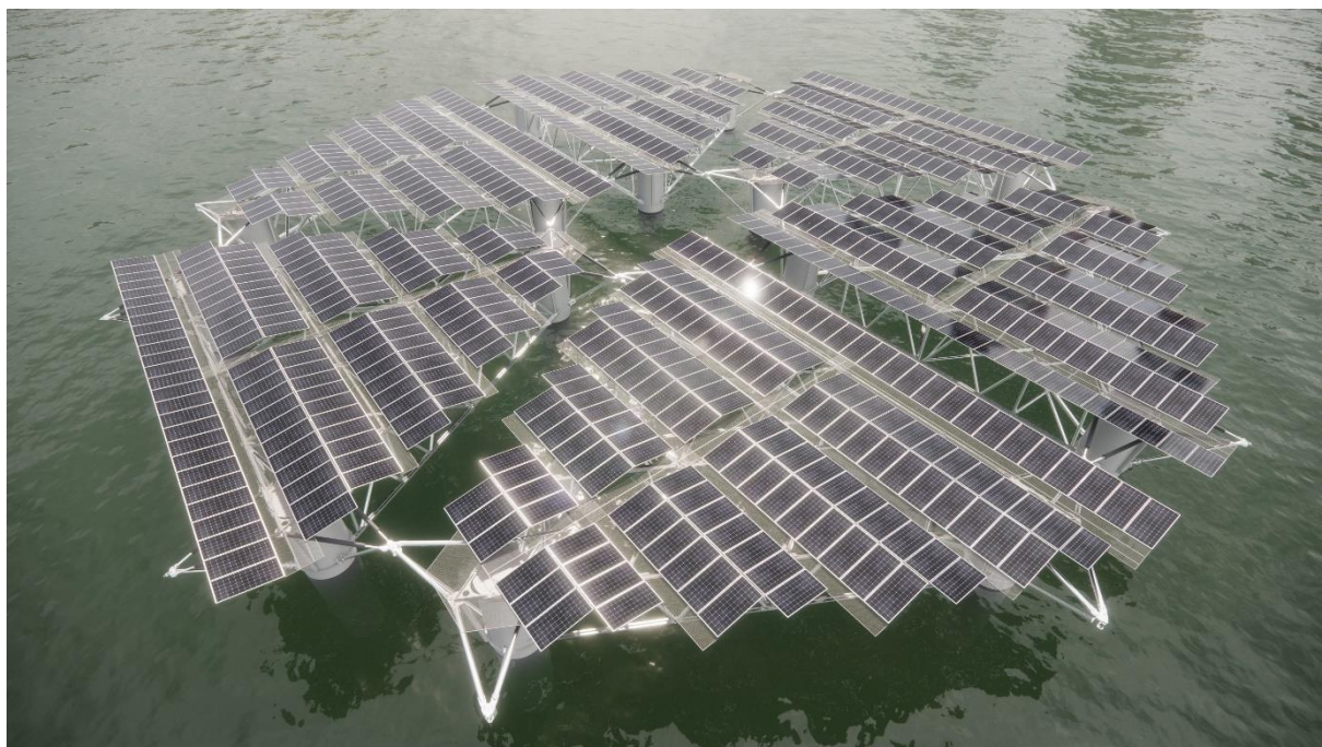
Caption: Close-up of floating solar power plant (credit SolarDuck)
